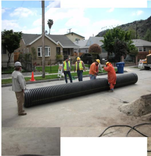
Parkway N4 bioretention area, with gravel bed ready to accept infiltration storage pipes
