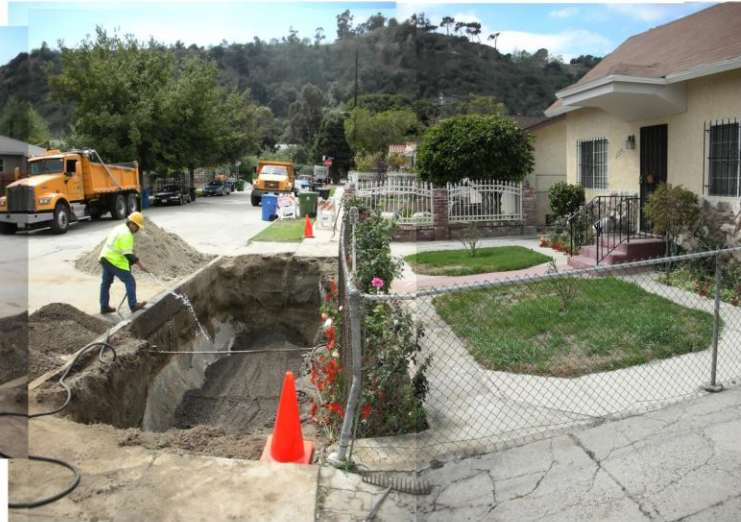
Parkway N4 bioretention area, with gravel bed ready to accept infiltration storage pipes
