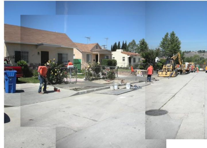
Parkway N4, with new driveway trench drains and walks in place ready for amendment and planting by NET
